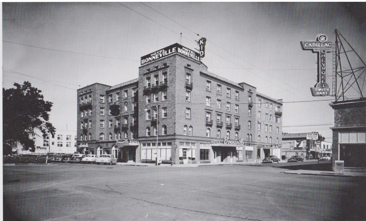
Bonneville Hotel 1951. Park and Constitution. The Cadillac and Chevy dealership is now the City Hall parking lot.
